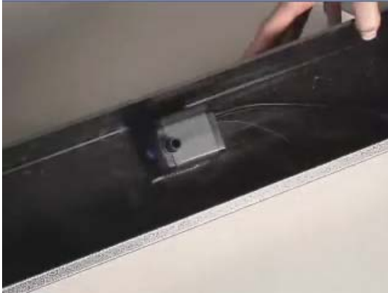
This is how the pump should rest in the tray. (Picture taken while tray is off the wall)
